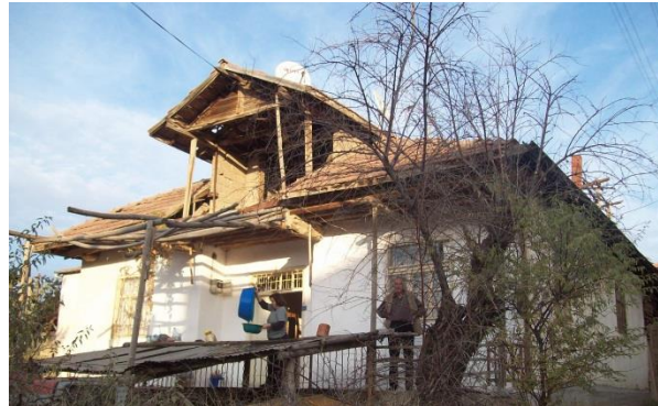
Figure 1. a “Poplar beam detail from Birgi/Izmir houses (19 th century).” b “Poplar branches used in wall masonry construction from Uçmakedere/Tekirdağ houses (19 th century)”. c. “Poplar beams and columns used in an adobe house in Hekimhan/Malatya (20 th century)”.
