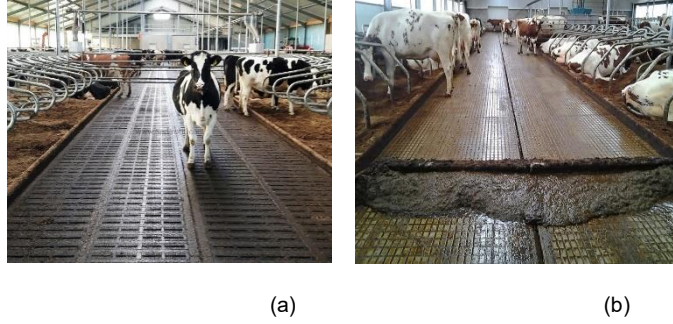
Figure 2. Slatted floors and scraper system application in barn.
